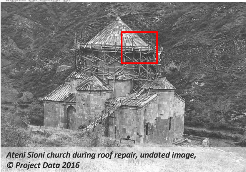
Reinforcement of roof exterior with cement, undated archival image
