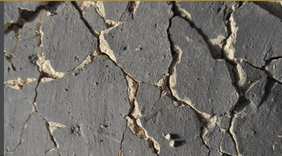
Face of the detached wall painting
