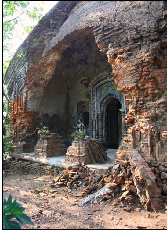
Plate 6: Present state of the temple façade
