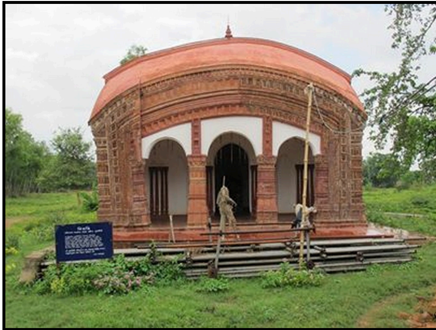
Plate 3: Temple façade after restoration by INTACH
