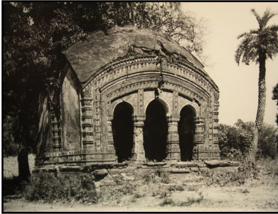
Plate 1: Dilapidated façade of the temple
