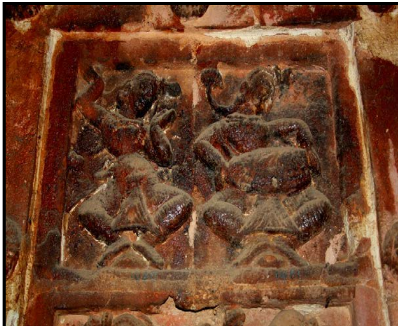
Plate 13: Deteriorated condition of terracotta plaques on the inner wall of Mandapa
