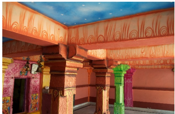
Fig 2: Sandblasted, Siddeshwara temple, Hollalagundi
